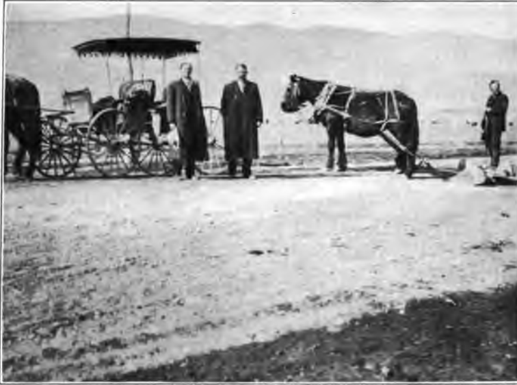
FIG. 11. CLOSE VIEW OF ROAD SHOWN IN FIGS. 9 AND 10, AND ALSO OF ROAD DRAG
